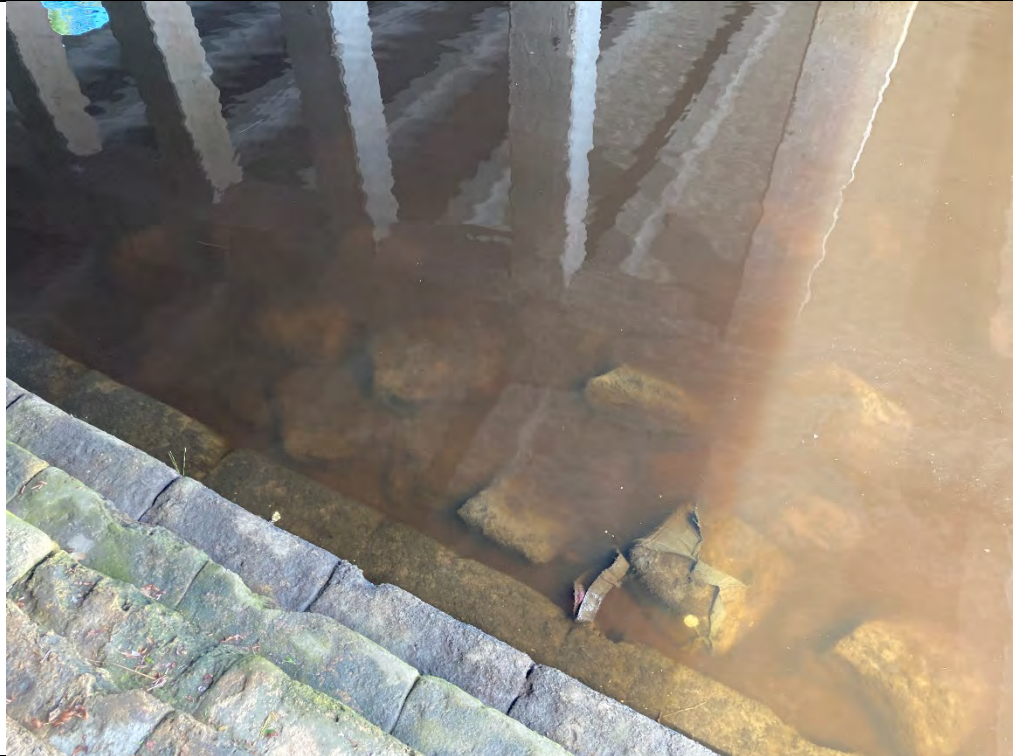
Picture 37: Riprap Right Abutment
