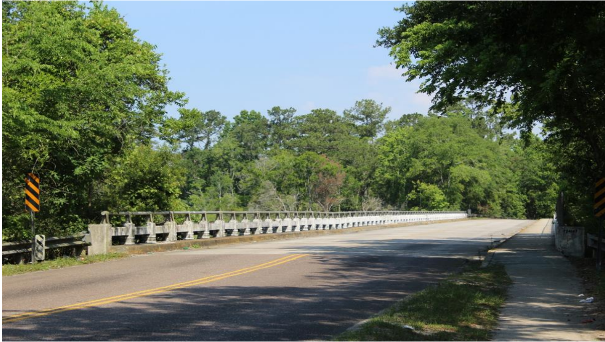
Ribault River Bridge, pre-construction
