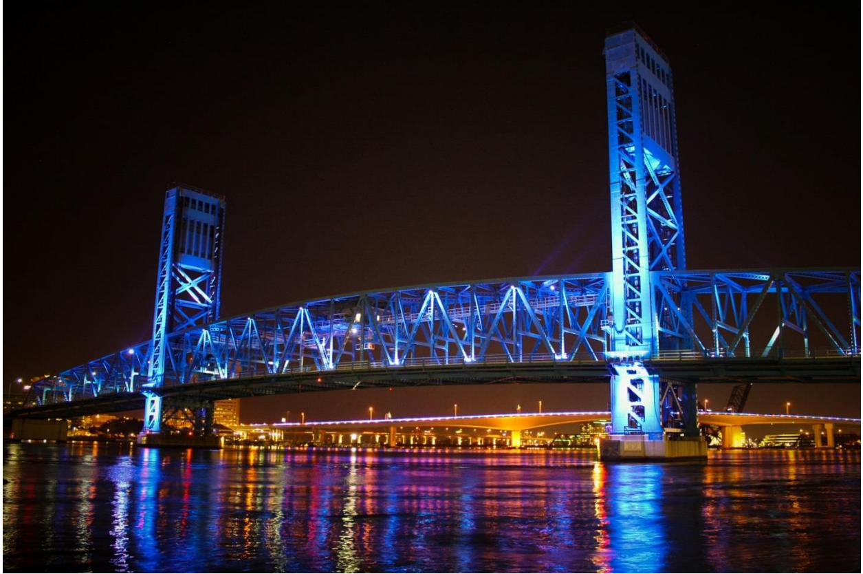
Main Street Bridge, Jacksonville, Florida
